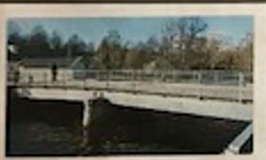
View of the southern part of Dämme bridge in Gothenburg.
